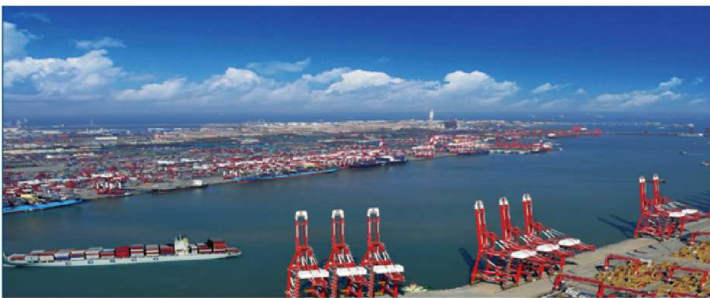
2016 the hot water reconstruction project of Qingdao port.
