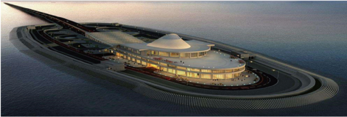
The artificial island hot water project of the Hong Kong-Zhuhai-Macao Bridge in 2019.
